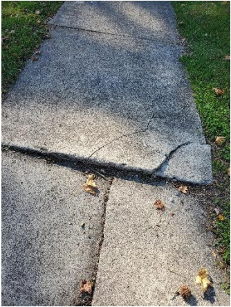
Fair : Uneven and distressed surface that hinders mobility of the average pedestrian. The sidewalk contains surface cracks, vegetation overgrowth, or debris.
