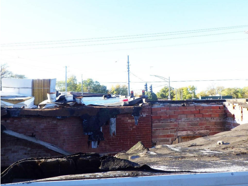
Image 5: Collapsed north roof – looking south.
