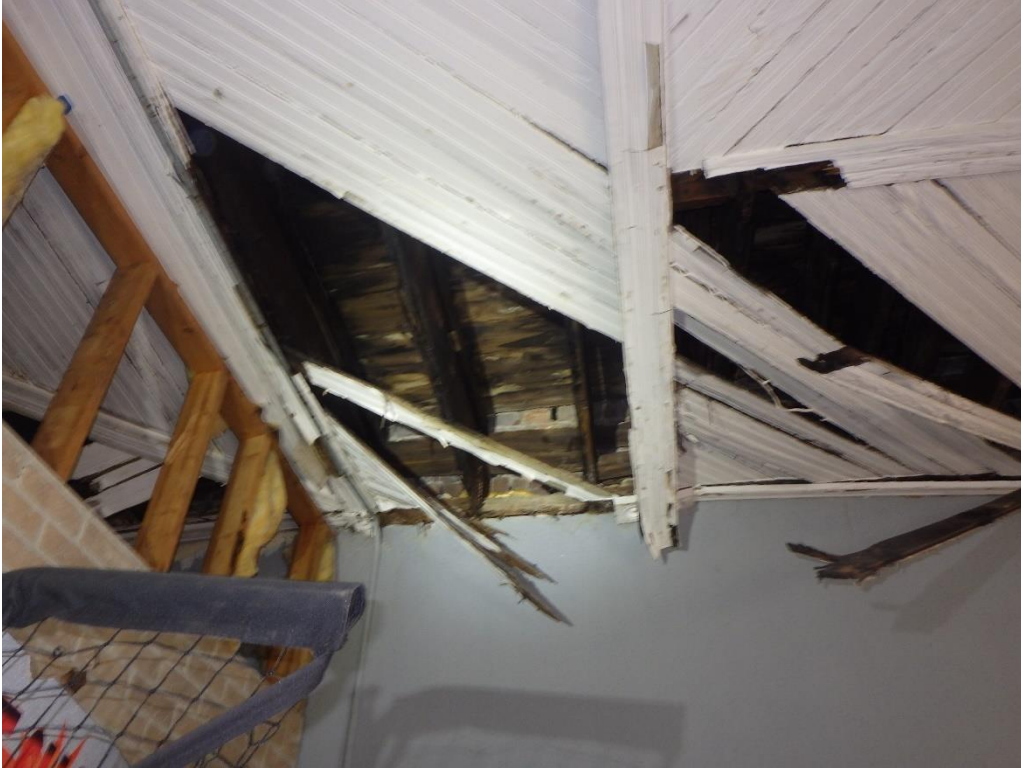
Image 12: Deteriorated ceiling/roof joists at east wall.
