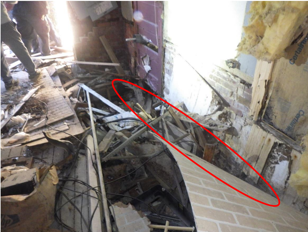
Image 16: East partially undermined wall.
