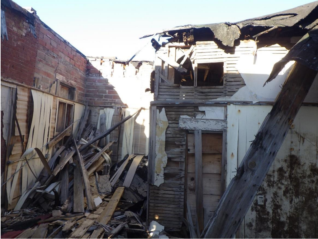
Image 17: Collapsed ceiling/roof at north structure.
