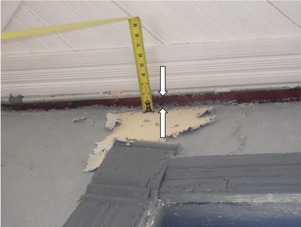
Image 9: Separation at ceiling along south wall.
