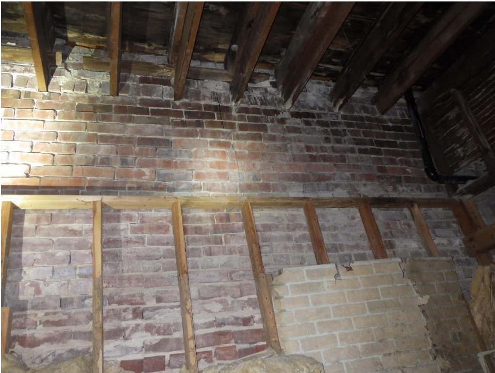
Image 13: Degraded condition of the west wall.
