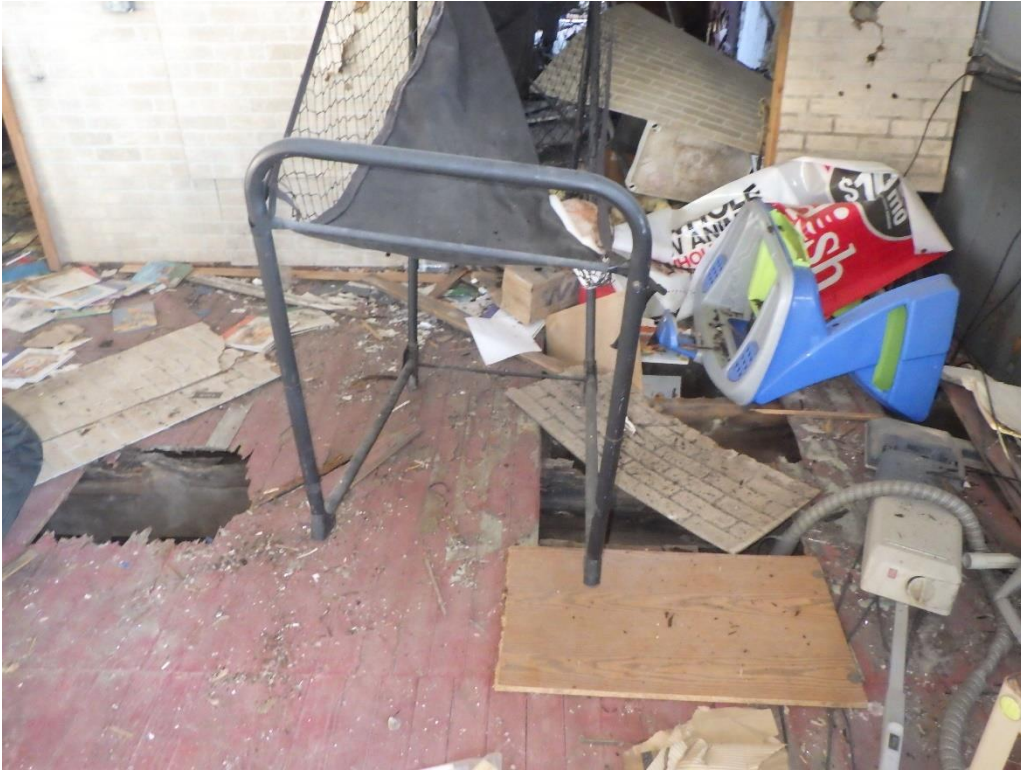
Image 11-A: Holes in the floor.
