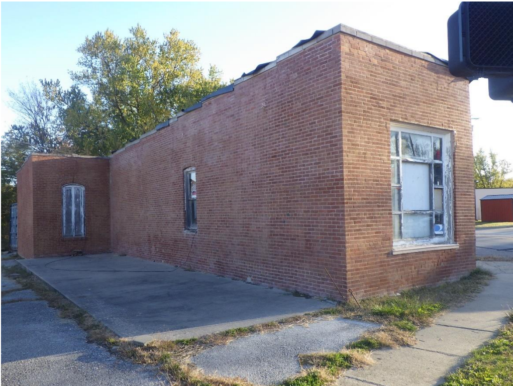
Image 4: Repointed exterior walls.
