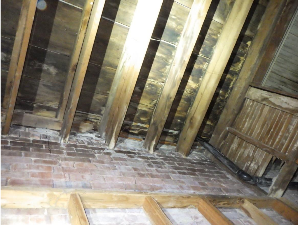
Image 14: Degraded roof sheathing along the west wall.
