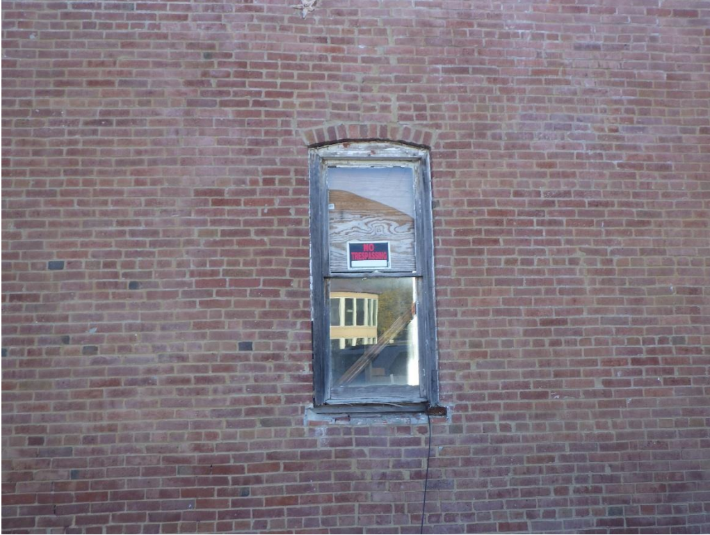
Image 1: Degraded west window.
