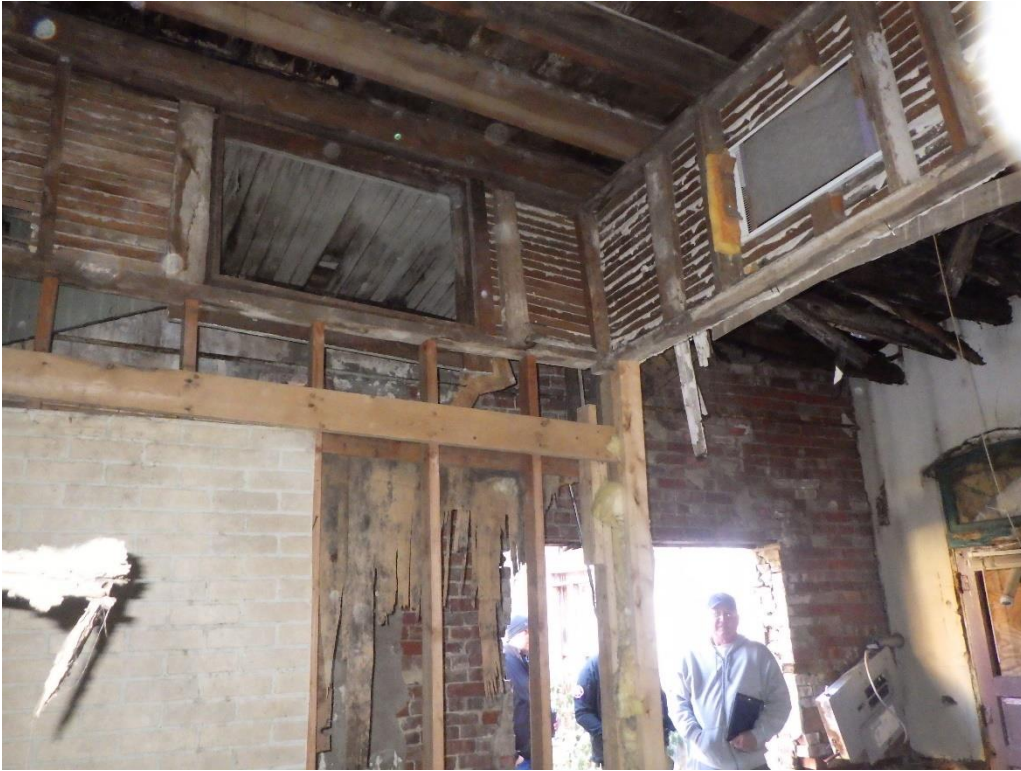
Image 15-B: Interior wall supporting the roof.
