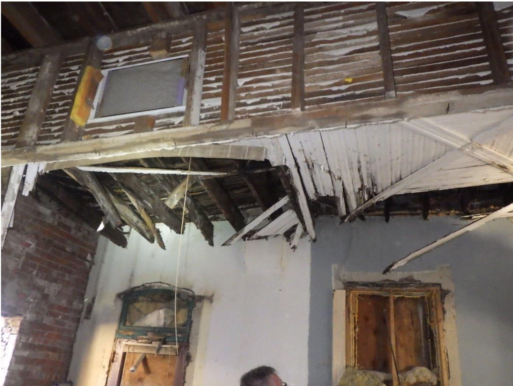
Image 15-A: Severely deteriorated joists along the east wall.
